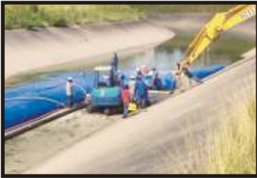
Concrete channel repair
