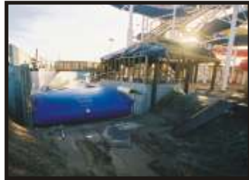
Water park construction & repair
